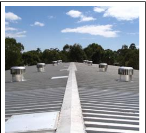
The ecopower EP600 has been used on Alexandria Hills State High School, to replace the existing spherical shaped wind driven ventilators as the system was not performing to desired standards.
